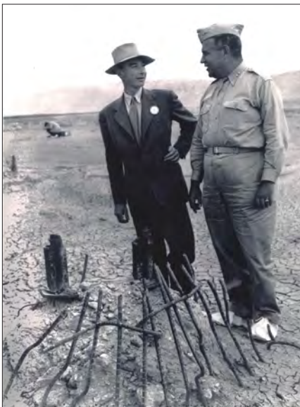
Figure 2: Photograph taken 20 July 1945 at the Trinity test site showing melted remains of the mostly vaporized 150 foot steel tower after detonation of the first atomic bomb. Present are two prominent test observers, physicist Robert Oppenheimer, who directed the Los Alamos Laboratory, and General Leslie Groves who served as the overall head of the Manhattan Project. Success of the test meant an atomic bomb using plutonium was feasible and could be readied for use by the U.S. military.
