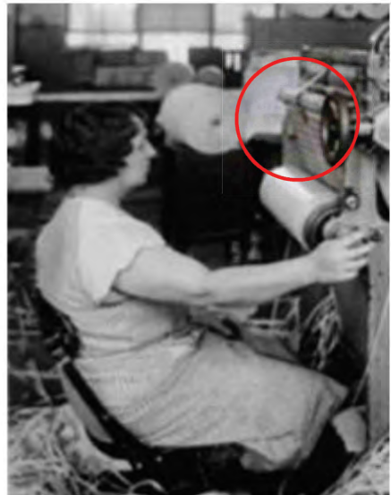
Figure 12: Front end of the perforator. Web alignment controlled by a metal pointer.
